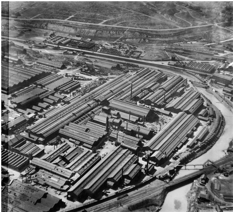
The East Heckla Steel Works in 1946 – now the site of the Meadowhall Centre © 1946 Reproduced by permission of English Heritage http://www.britainfromabove.org.uk/image/eaw000811
