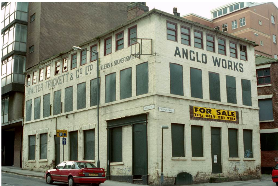
The Anglo Works in Sheffield, one of a small number of surviving city centre cutlery and silversmith factories.
