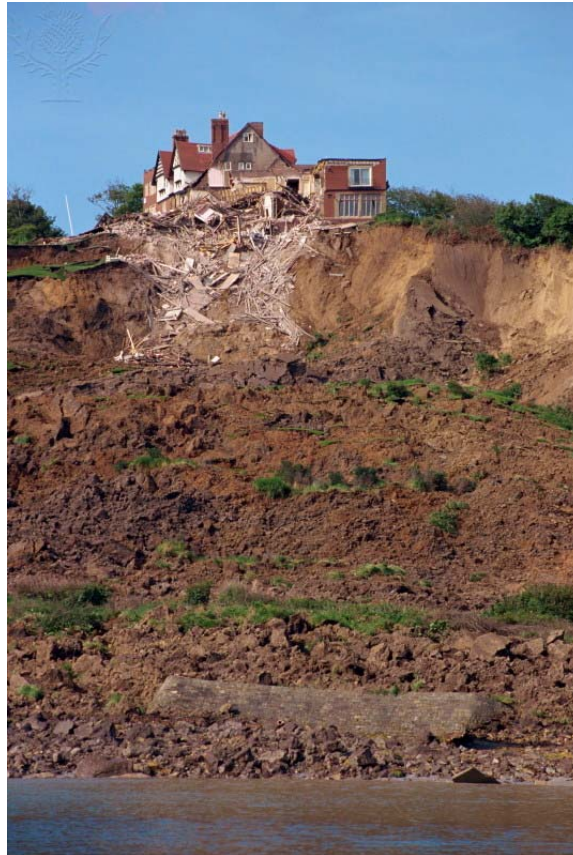
Landslide taking part of the Holbeck Hall Hotel down 30m clay slope on 6th June 1993, Scarborough, Yorkshire, England
