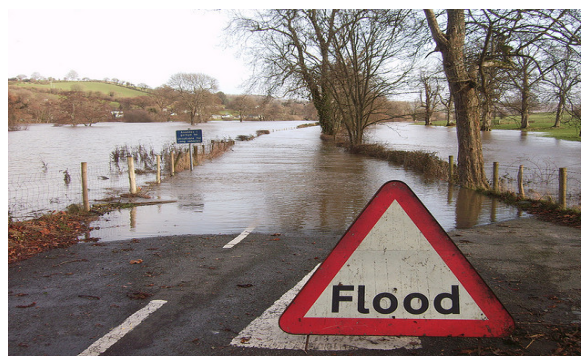
Flooded road in Wales
